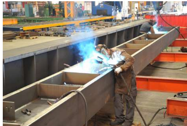
Fit Up and Welding
